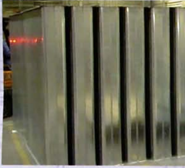
Slide-in baffles for existing ductwork
