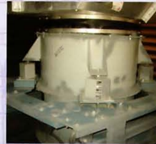
Flex Connections and Isolation
