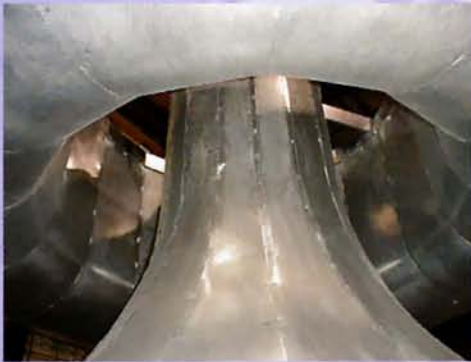
Inlet view of a Radial Inlet Silencer (RIS).
