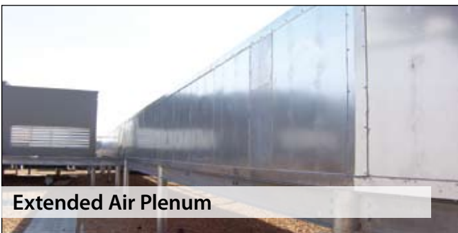
Supply Air Discharge Plenum
