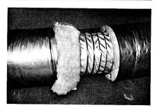
4) Peel back vapor barrier and insulation again approximately three inches each side of joint. Tape core with two wraps of tape, each wrap overlapping previous wrap at least 25% and following natural path of duct helix.
