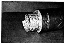
3) Screw second core inside first three full turns. Check that helix of inside core tracks properly into helix of outside core without crossthreading. Pull joint lengthwise to take up slack. If insulations will not butt together, screw in further until insulations butt.
