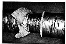
Fold insulation and vapor barrier back over core joint. Tape barrier with two wraps of duct tape lapped approximately 25%. An approved clamp may be used in place of or in combination with the duct tape.
