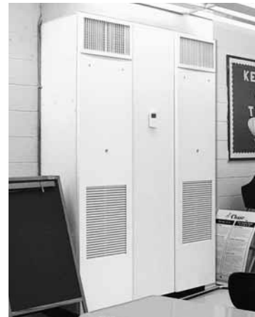
Custom side-by-side exposed installation
