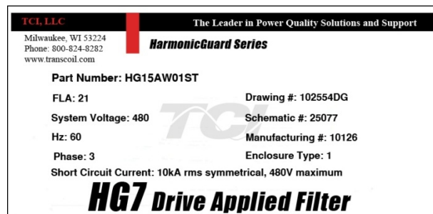
Figure 1 – Typical HG7 Harmonic Filter Nameplate
