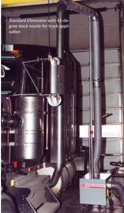
Basic/Base Plate Eliminator for truck application - attached to overhead exhaust system
