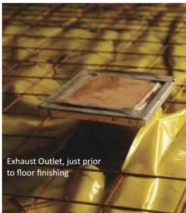
UnderDuct-VE System used in service facility
