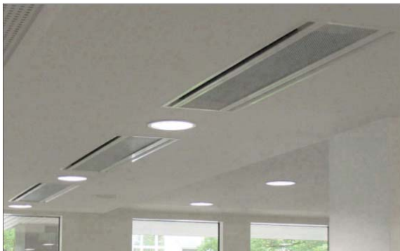
Installation in plasterboard ceiling
