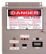
High Voltage Power
